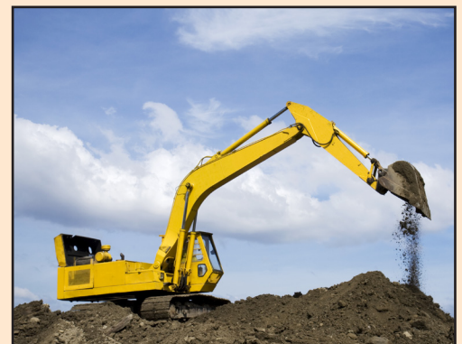
Heavy equipment excavating
