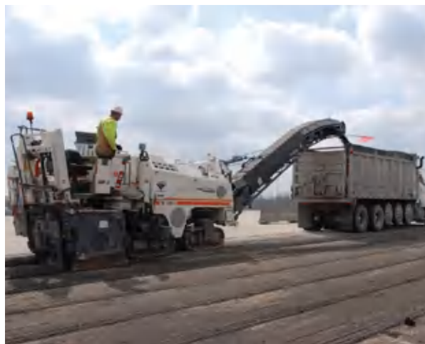
Milling machine milling asphalt road and loading debris into haul truck.
