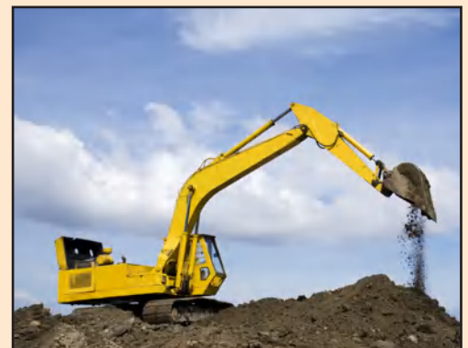
Heavy equipment excavating
